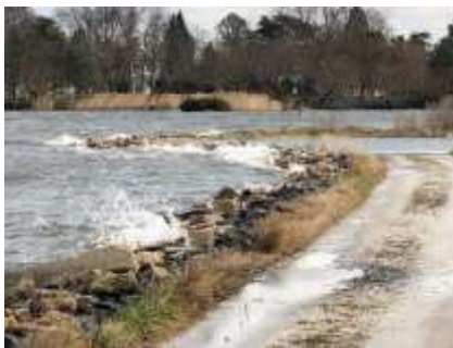
Parking Lot..... is under water.
